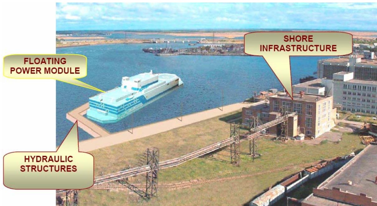
Fig. 1. General view of NPP.
